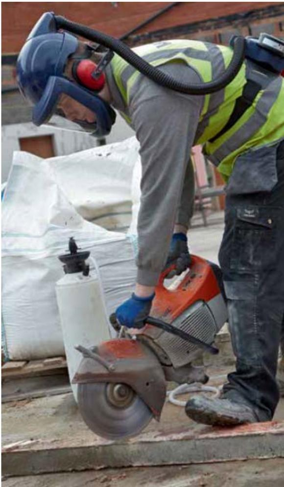
If this is the case, then the only alternative is to use a positive pressure respirator as illustrated, which doesn't rely on the seal and will still give you adequate protection.
