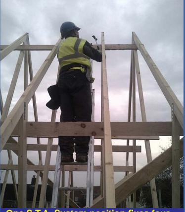
One S.T.A. System position fixes four trusses (two trusses on either side of the ladder)
