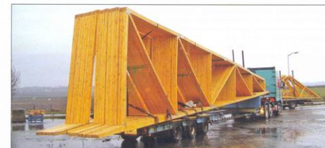
Sites should provide a strong, level surface and appropriate equipment for unloading
