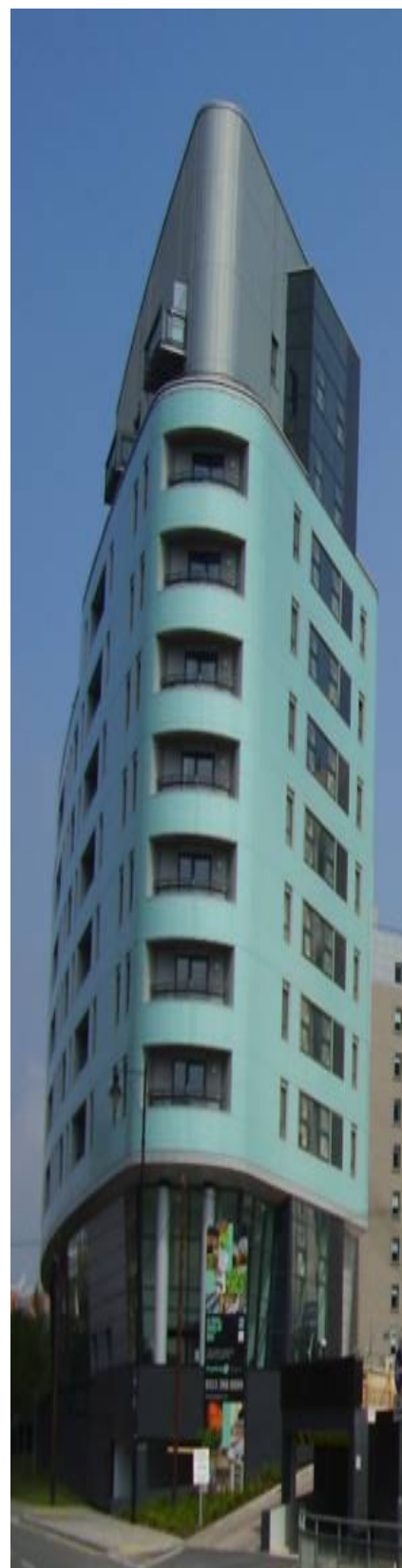
Source: DTZ photos: The Gateway
