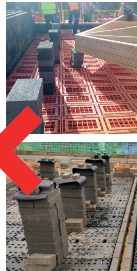
Above left - Good practice: system loaded out over the vertical posts, uniformly distributed and within the load limit as set by the manufacturer.
