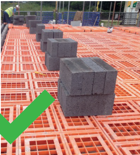
Above left - Good practice: system loaded out over the vertical posts, uniformly distributed and within the load limit as set by the manufacturer.
