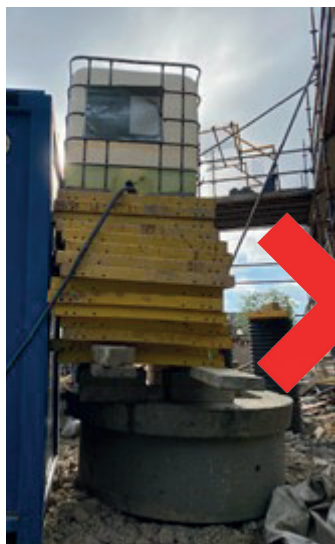
Above left - Good practice: system loaded out over the vertical posts, uniformly distributed and within the load limit as set by the manufacturer.
