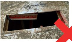
Below: Bad practice - an operative was seriously injured when he stood on the removed section of the floor, causing the hatch to dislodge and he fell to the floor below.
