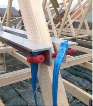
Two photographs illustrating roof truss construction. The top photograph shows a worker in a high-visibility vest standing on a wooden truss structure, likely performing bracing or access work. The bottom photograph is a close-up of a wooden truss joint, showing a metal plate and a blue ratchet strap used for securing or bracing the structure. |
