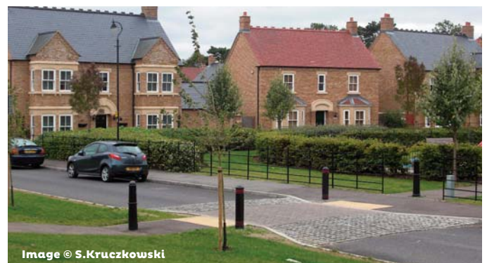
At Fairfield Park in Bedfordshire, vertical calming and 'pinch points' remind drivers they are in a 20mph zone
